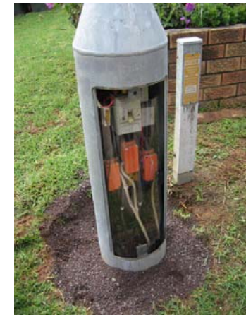
When finished work on column, fold sheet flaps back inside hatch and tuck Velcro out of way.
