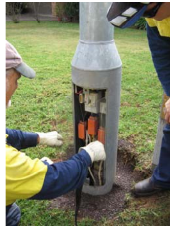
Insert sheet along inside wall of column pushing past any internal resistance.
